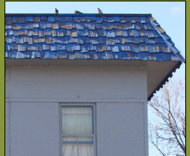
Before Picture of Large Renovation Project in Red Deer
